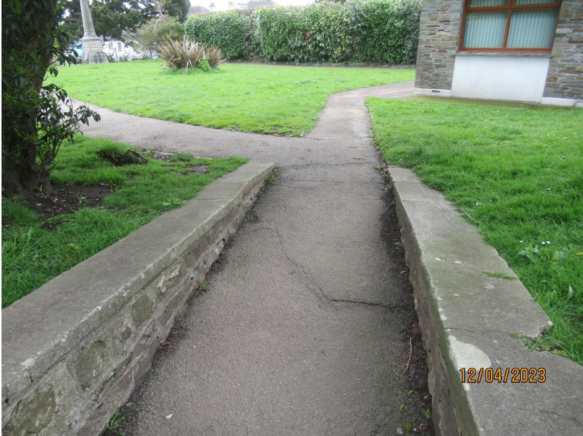
P18 – north-west corner footpath
