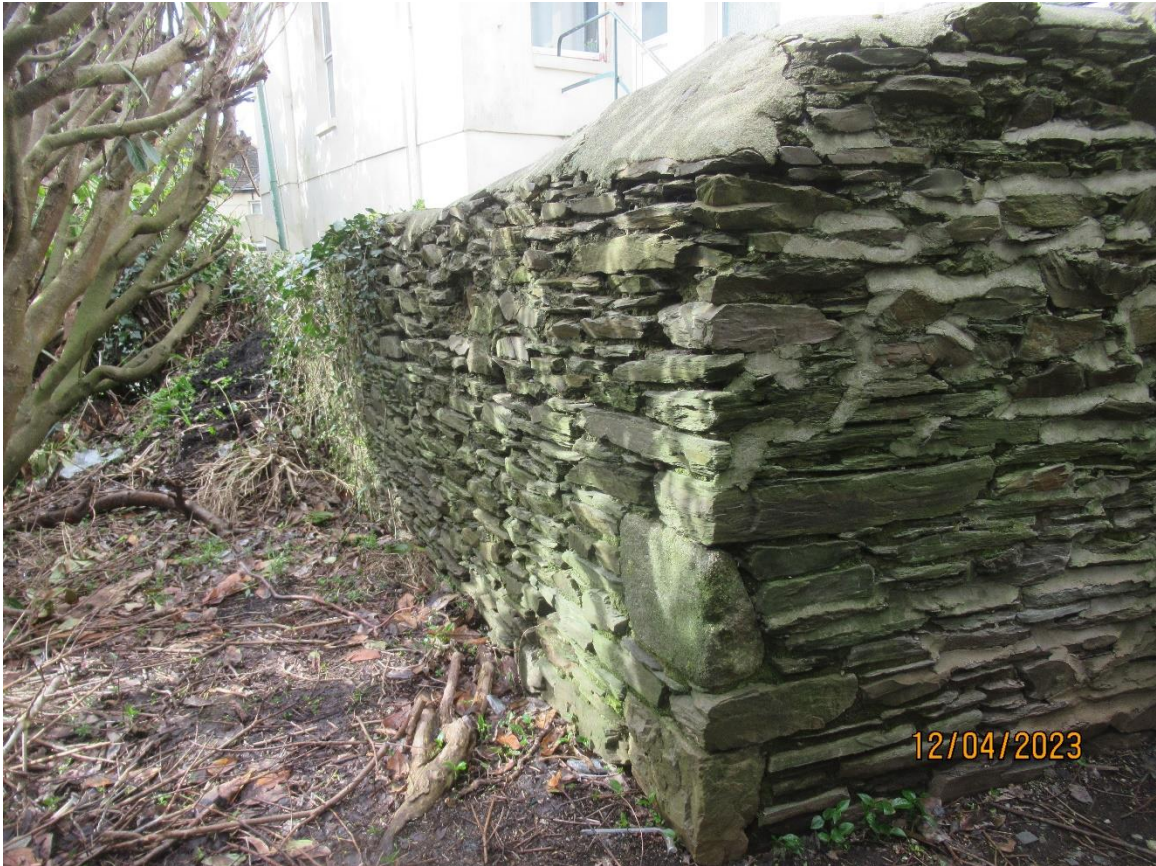
P7 – west boundary wall
