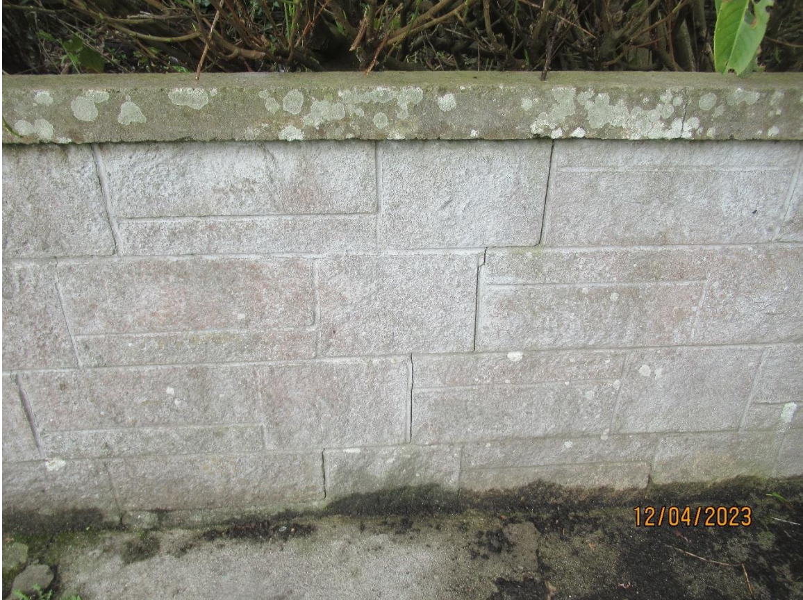
P22 – walling to bandstand
