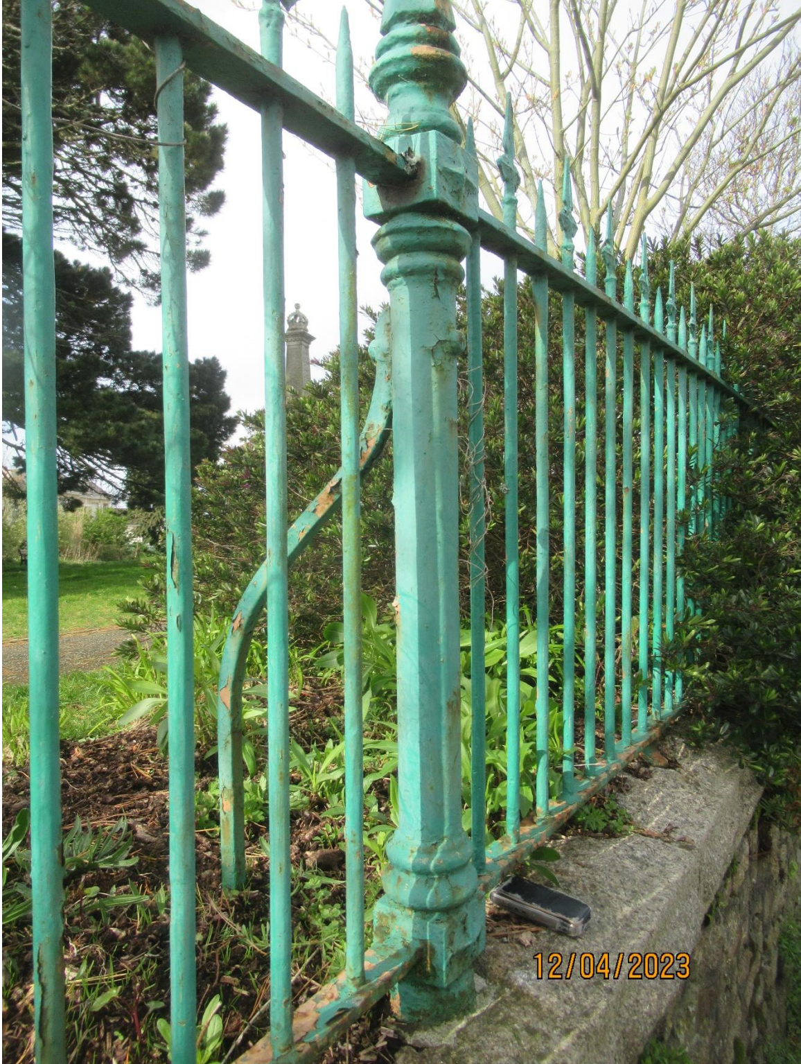
P13 – East length of Callington Road railings
